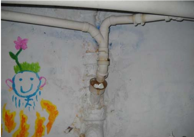
Photograph No. 45 Typical waste piping in the basement of Baxter House.
